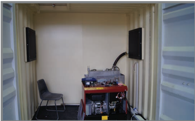
Container fit out
